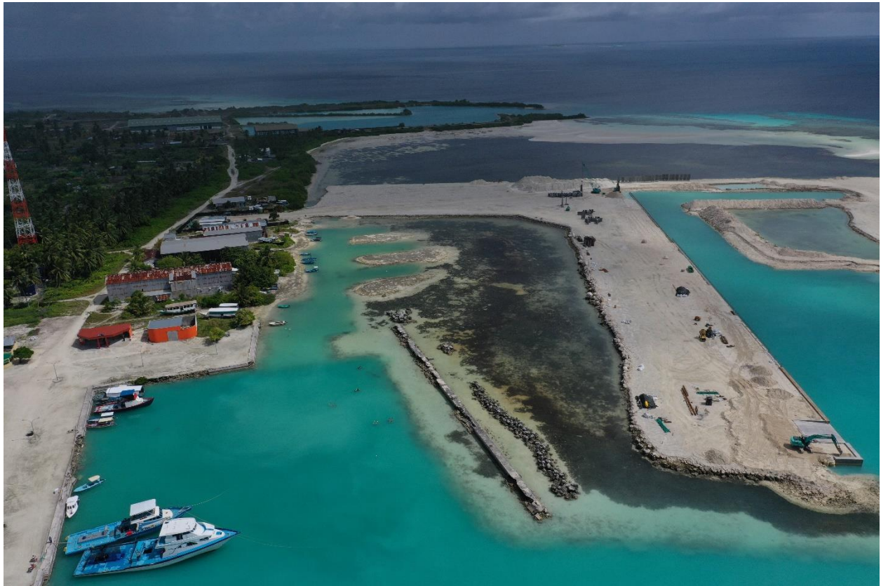
Figure 107 New Harbour Construction progress indicating large changes in the shoreline of the island
